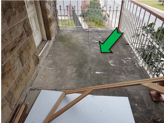
Photo 1. Exterior, level one, verandah, floor – non asbestos-containing compressed cement sheeting.
