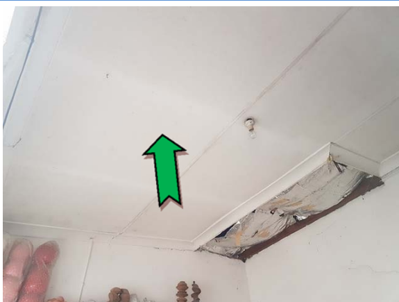
Photo 5. Interior, shed, ceiling, throughout – non asbestos containing fibre cement sheeting.
