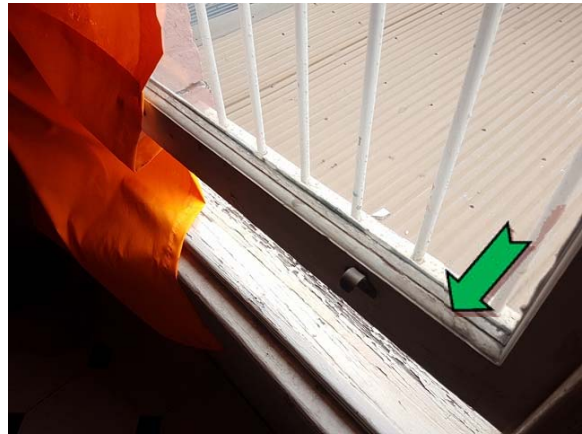
Photo 4. Interior, window frames, throughout – non asbestos-containing window caulking.
