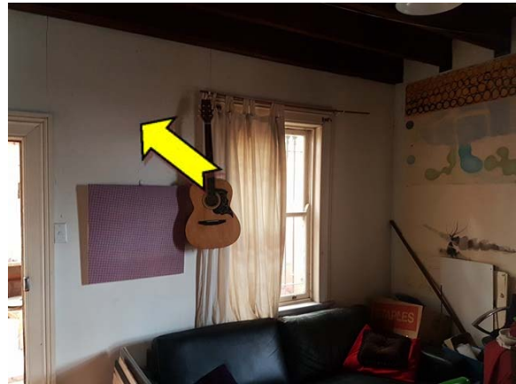
Photo 16. Interior, ground level, walls – suspected lead-containing white upper paint systems.
