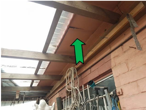
Photo 3. Exterior, shed, eaves – non asbestos-containing fibre cement sheeting.
