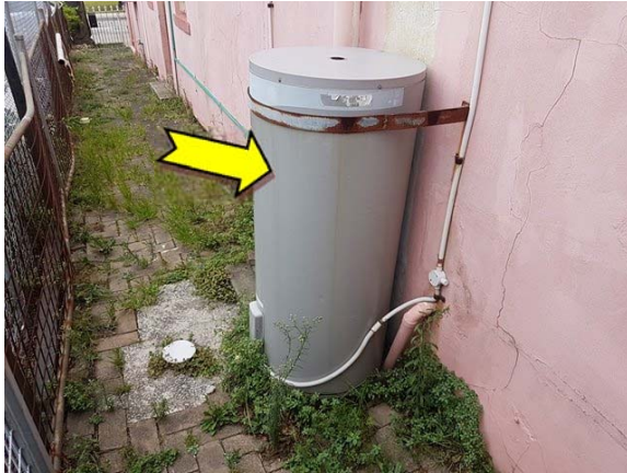
Photo 7. Exterior, east elevation, hot water heater – suspected SMF internal insulation material.
